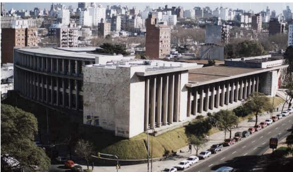
School of Architecture, Design and Urbanism (University of the Republic - Uruguay), designed by Fresnedo Siri and Muccinelli in 1946.
